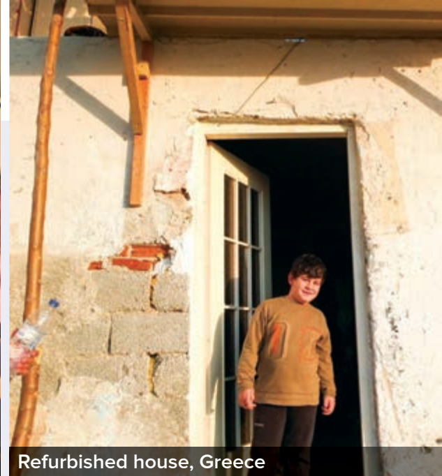
House repair, Greece
