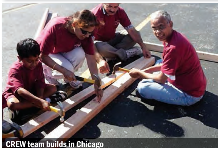
Building homes in Chicago
