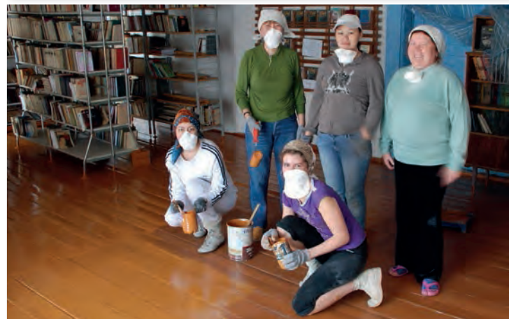
Volunteers perform building repairs, Kazakhstan
